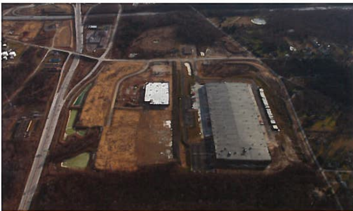
On left, is Costco Wholesale Club; and to the right, is Arhaus Distribution Center and Headquarters.
